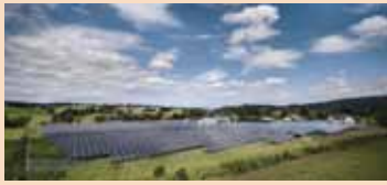
Solarpark in Eschenburg-Hirzenhain
